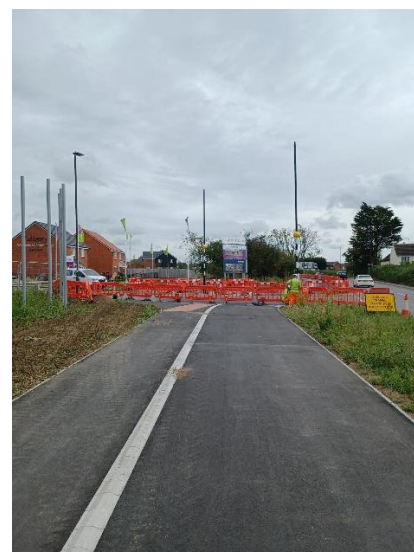
Phase 3A – Belisha beacon installation at Goldsmith Road works
