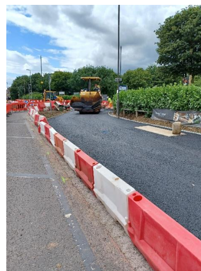
Phase 2B – Surfacing works at Brickhampton Golf Course
