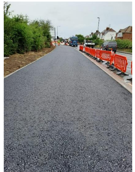
Phase 3A – Surfacing works
