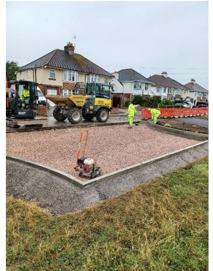
Phase 1B - Dancey Road turning circle surfacing preparation
