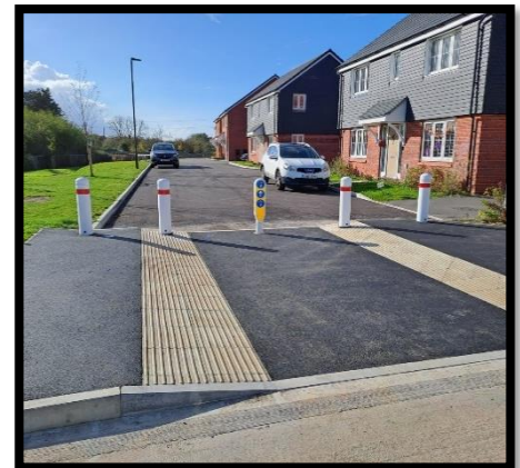
Phase 3A Dancey Road bollard installation
