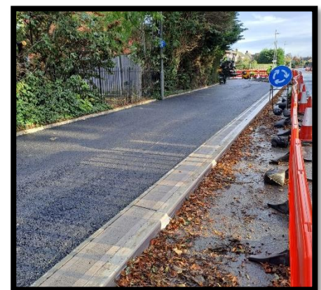
Phase 4B Base layer surfacing
