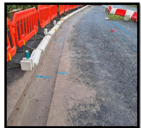
Phase 2B Demarkation kerb installation
