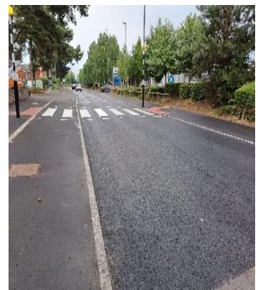
Phase 1B - Tabletop road crossing outside Tesco
