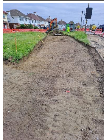
Phase 3A – Footpath and cycleway formation works
