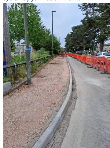
Phase 1B- Westbound ready for final surfacing
