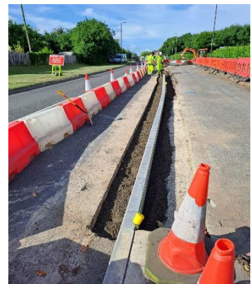
Phase 2B – Kerb installation Brickhampton Golf Course
