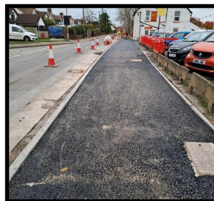
Phase 2B surfacing works
