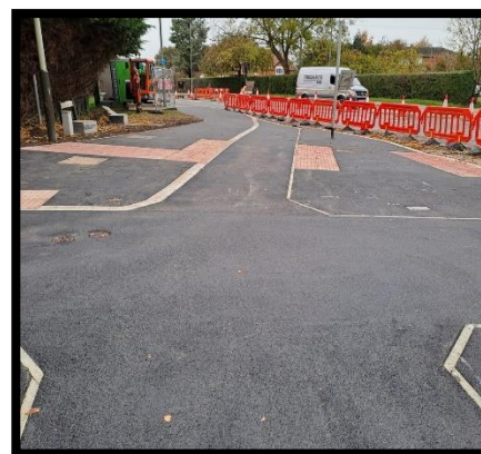
Phase 4B NW corner surfacing complete
