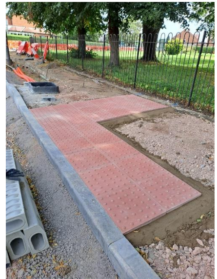
Phase 3A – Surfacing works
