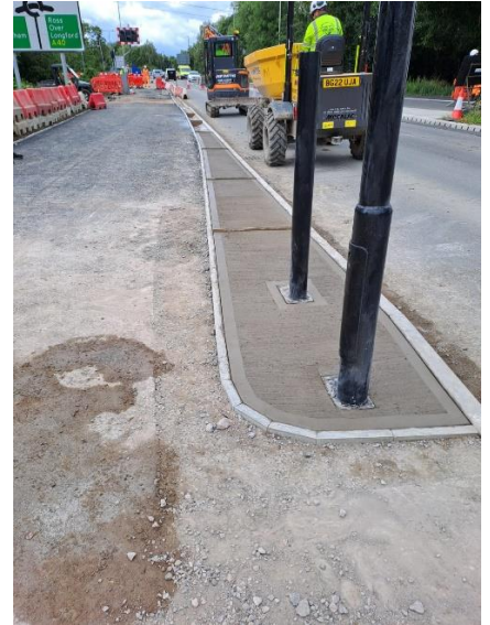
Phase 4A - Buffer zone and carriageway kerbs complete
