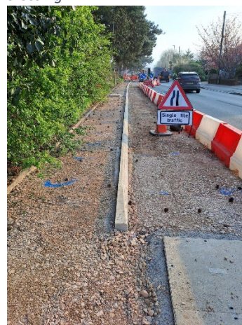
Phase 2A ready for surfacing
