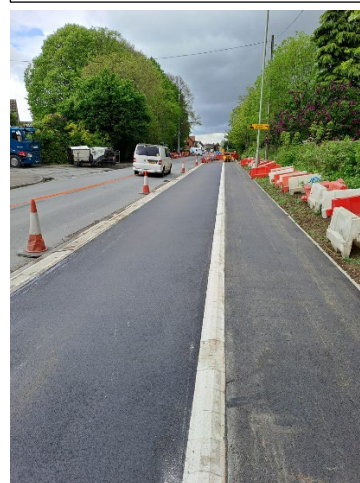
Phase 1B – Surfacing Complete
