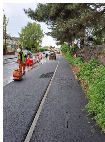
Phase 2A - Surfacing
